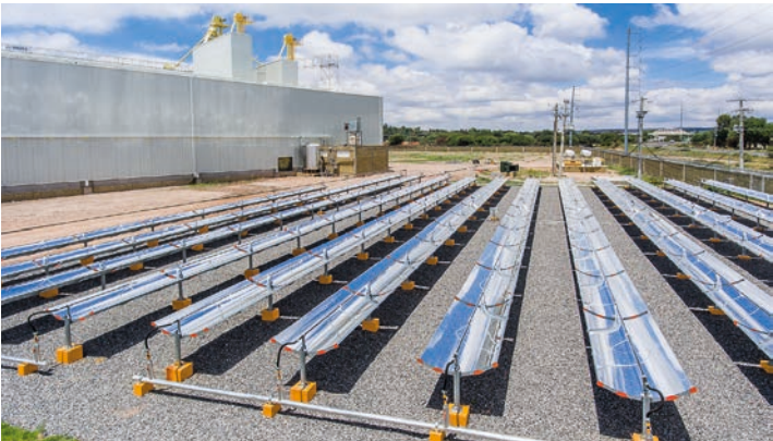
Parabolic trough collectors installed at Comercial Forrajera de Lagos (COMFOSA) in Mexico
