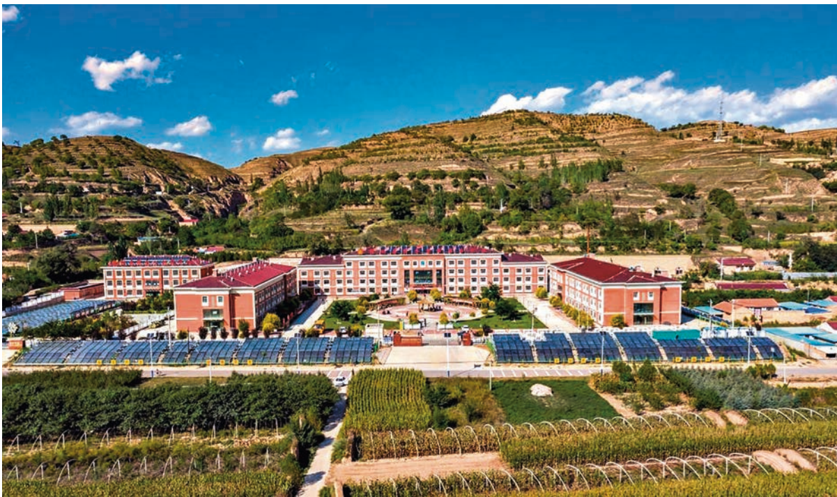
Solar combi-system consisting of flat plate collectors and a heat pump for space heating at a nursing home in Guyuan County, Ningxia
